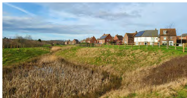
Figure 22: An attenuation pond which forms part of the SuDS strategy for part of a new residential development within the west of the Neighbourhood Plan Area.
