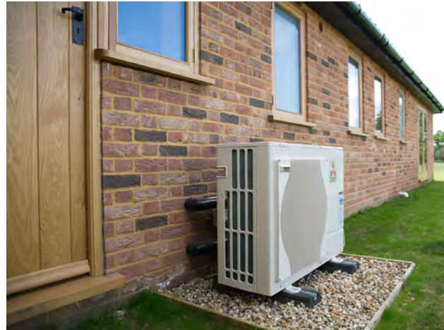
Figure 77: Air source heat pump unit located to the rear / side elevation of a dwelling, so to avoid its visual impact on the dwellings frontage and wider streetscape
